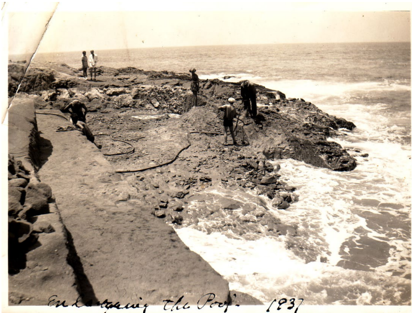
Figure 26: Tidal Pool under construction, view west (Braff/Christou Collection, 1937)
