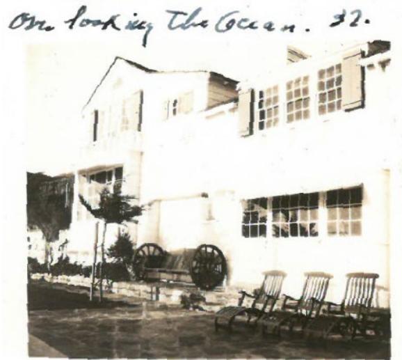
Figure 18: West elevation of Main House, view northeast (Braff/Christou Collection, 1932)
