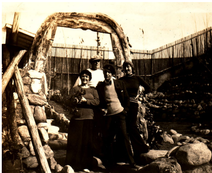
Figure 16: Wooden arch at subject property, view east (Braff/Christou Collection, c. 1930s)
