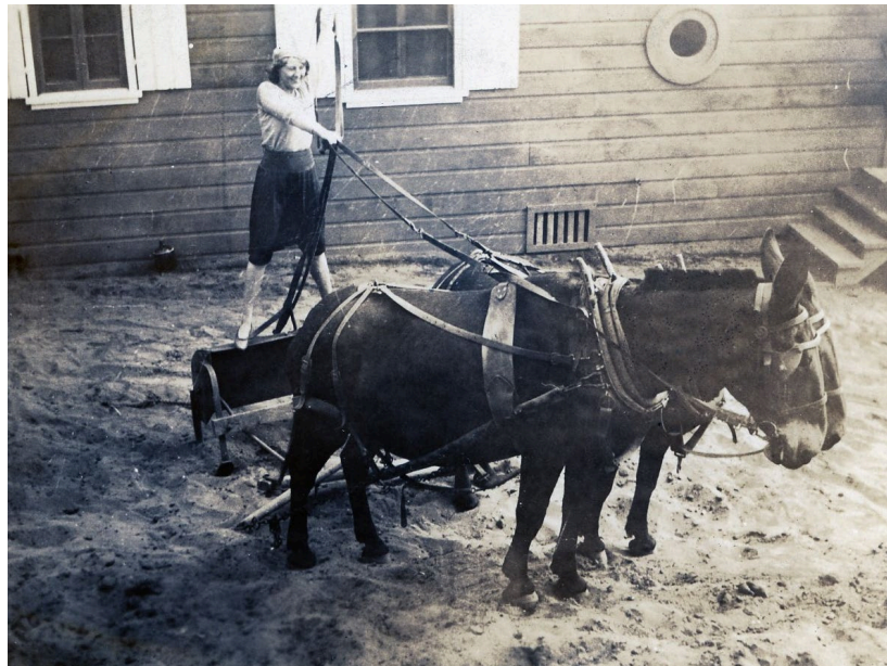
Figure 13: Main House, north elevation, view south (Braff/Christou Collection, c. 1927)
