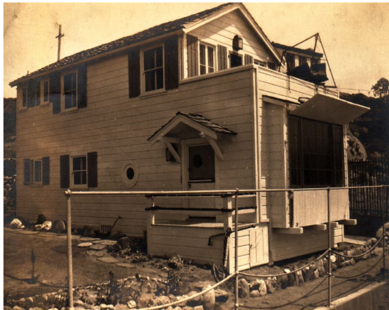
Figure 14: Main House under construction, north (left) and west (right) elevations, view southeast (Braff/Christou Collection, c. 1927)
