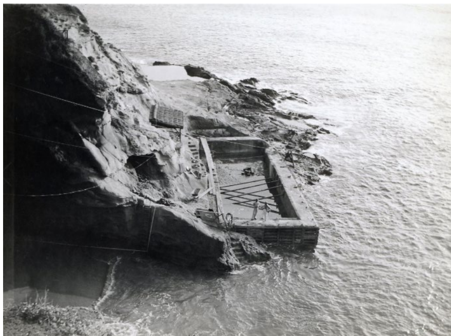
Figure 27: Tidal Pool under construction, view west (Braff/Christou Collection, 1937)
